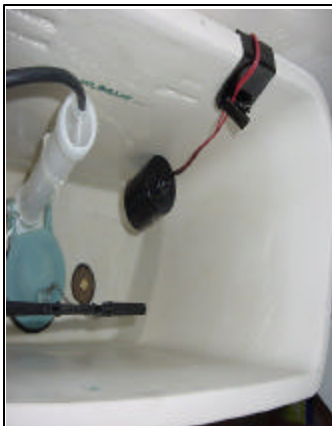
Figure 1: Aluminum Clip location Figure 3: Flush Counter set-up
