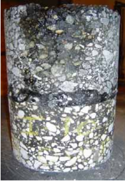
Figure 3-3. Cored Mixture in Cracked Section
