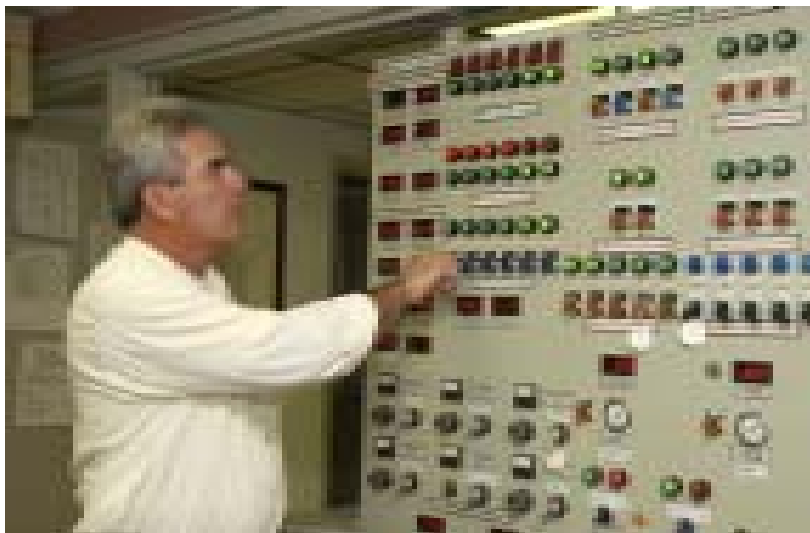
Left: Plant operator Gary Bittner looks over the equipment control panel.
