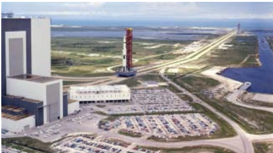
ON MAY 20, 1969, the vehicle, mobile service structure and mobile launcher began traveling along the crawlerway to the launch pad. Once at its launching destination, the processing didn't stop.
