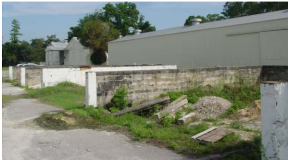
Storage Bins Located Next to Building #1622
