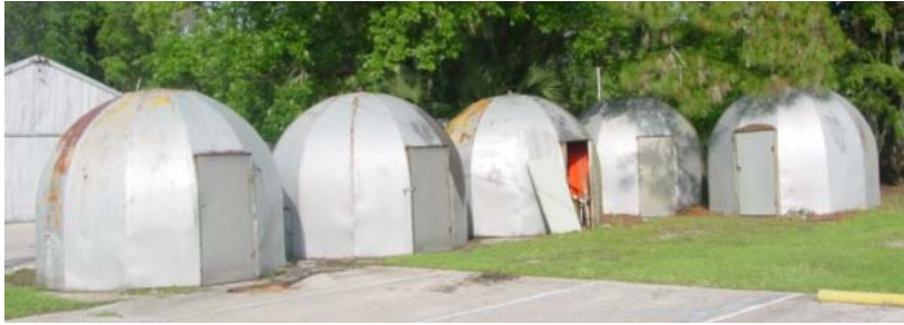
Storage Pods Located Next to Building #1607
