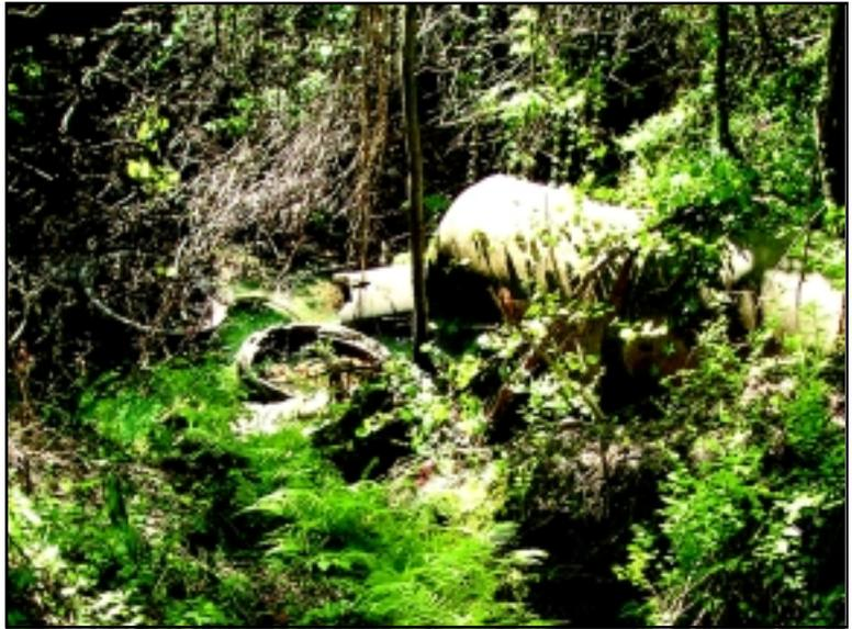
***Decades-old stormwater conduits, exposed by constant erosion, crumble into a small runoff pond located in a ravine behind Mechanical Engineering. The ravine has been designated a conservation area and the conduits are scheduled for eventual removal.***
