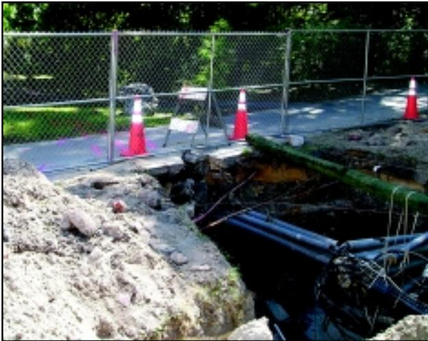
**An excavation near the Reitz Union reveals underground telecommunications lines. The old manhole in this spot is being replaced, as it had become too small to effectively service the constant growth of the utilities network in the area.**
