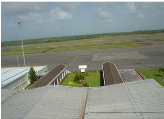
Photograph 1-8: CJIAC International Airport
