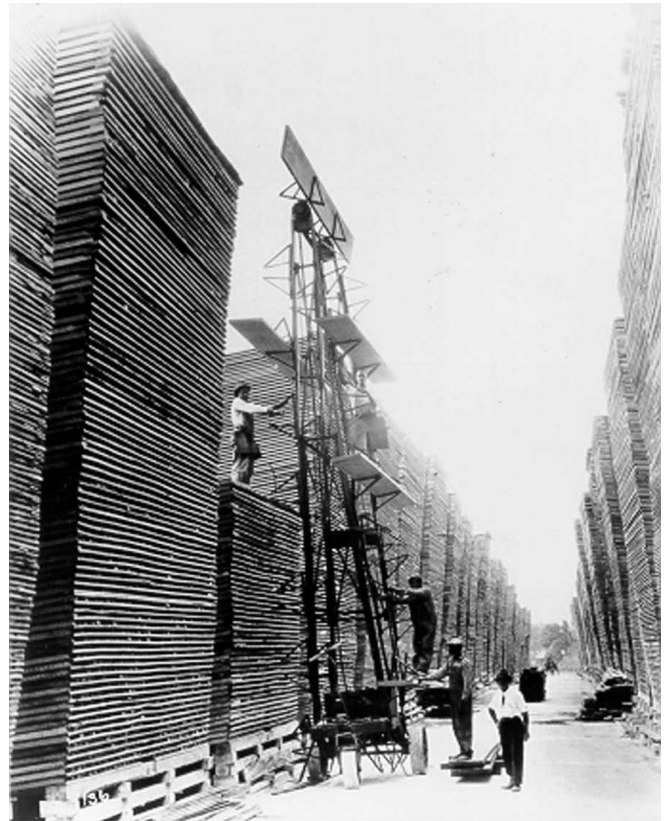
Figure 14. A typical cypress yard and stacking machine.
