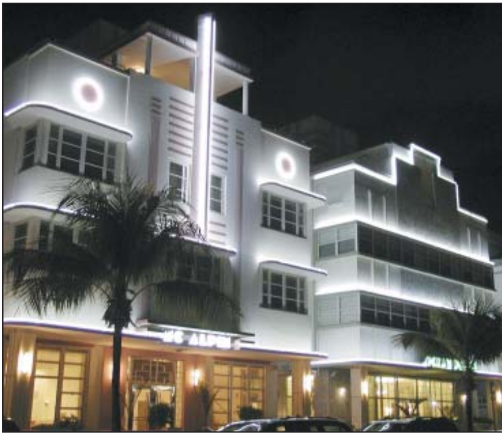
Art Deco on display: Neon lighting was important feature of Art Deco because it became part of the architecture.
