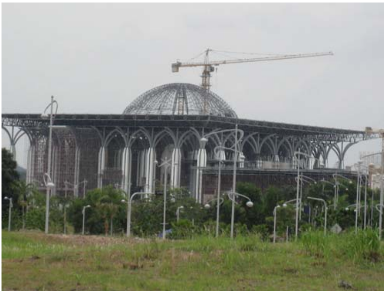
Figure 4-27 The National Mosque, under construction. Author 2008.
