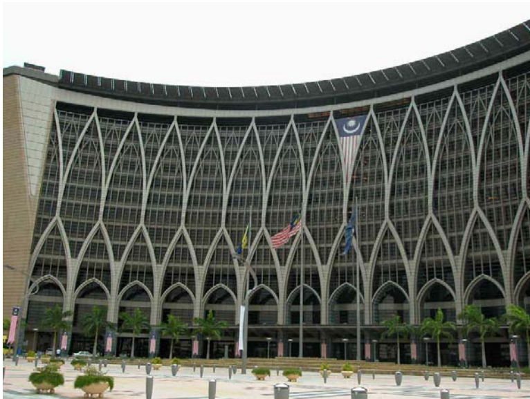
Figure 4-14. Ministry of Finance building. Author 2008.
