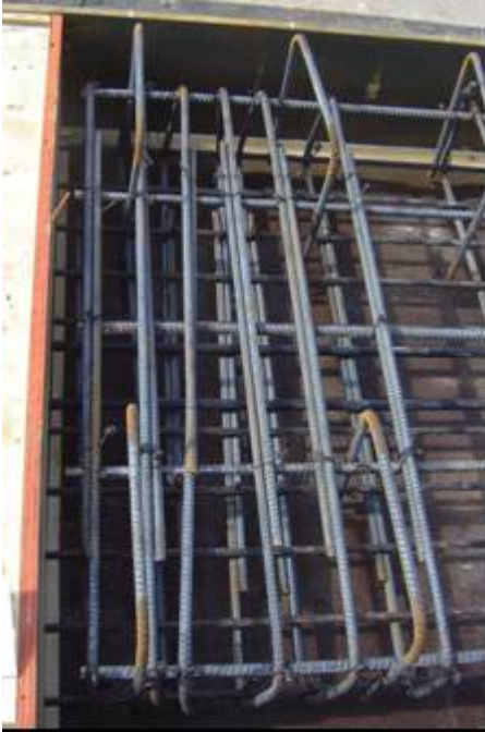
Figure 16. Reinforcement at end of flat slab
