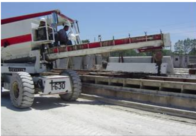
Figure 19. Casting of flat slabs
