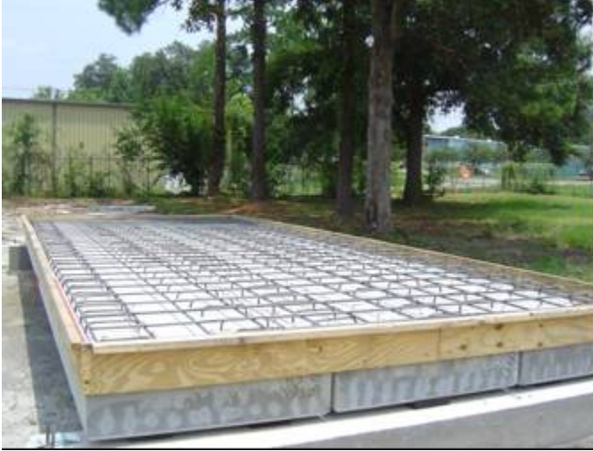
Figure 25. Reinforcement and formwork on precast slabs before topping placement
