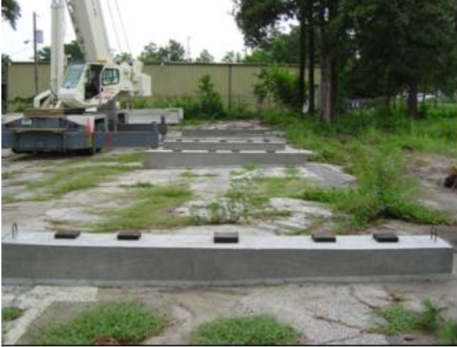
Figure 22. Concrete supports with neoprene bearing pads before placement of precast slabs
