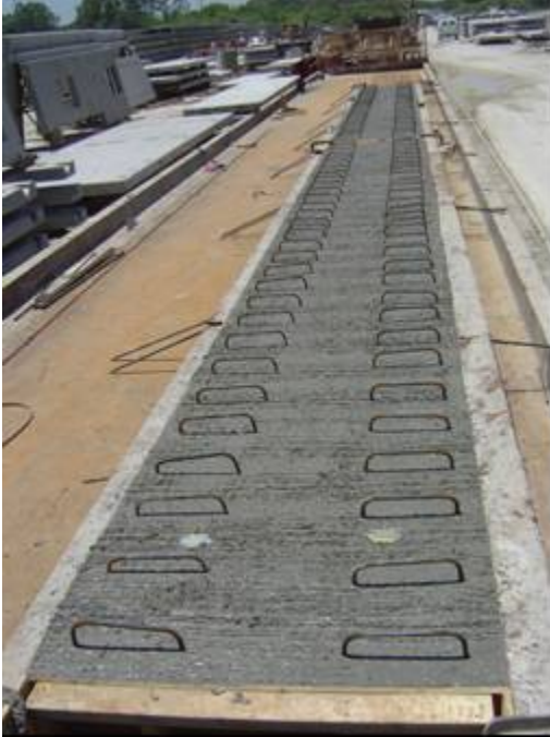
Figure 20. Finished flat slab with hoisting anchors installed
