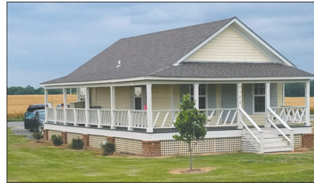
A view of the exterior of what Little Custom Homes plans to make. [PHOTO COURTESY MERCER ASSET PARTNERS]
