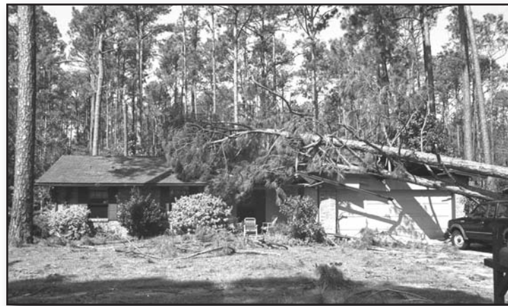
Hurricane Opal was a Category 4 hurricane that caused severe damage along the northern Gulf Coast of the U.S. in October 1995. Here, a storm-toppled tree on a house in Niceville.
