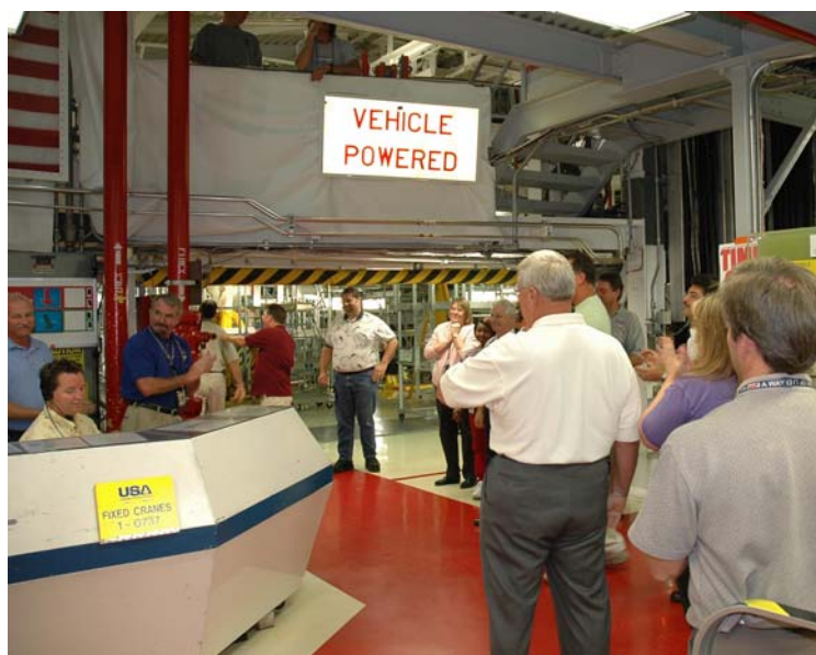
IN ORBITER Processing Facility bay 2, workers applaud as the orbiter Endeavour's electrical system is partially powered up after nearly two years. Endeavour's orbiter major modification period began in December 2003.
