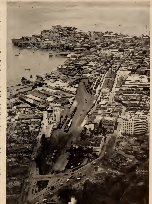
The Panama City railroad yards and buildings will be transferred to Panama as soon as freight and passenger facilities are established within the Zone.
