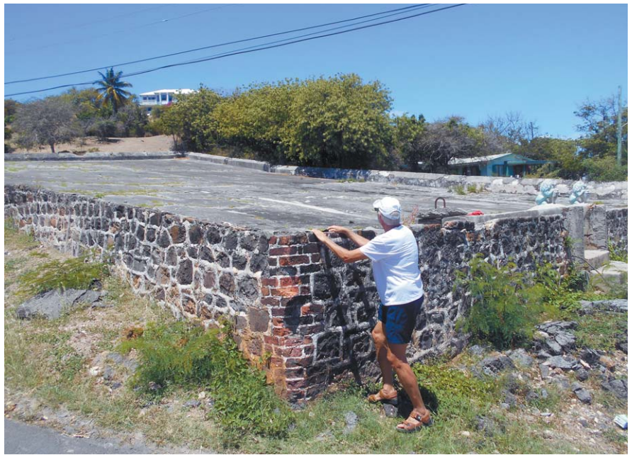
Not far from the main road to Nelson’s Dockyard there is an old water catchment, surrounded by a low wall. This is your destination
