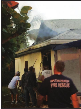
Members of HTVFR move in to assess damage. Photo: Troy Pritchard.
