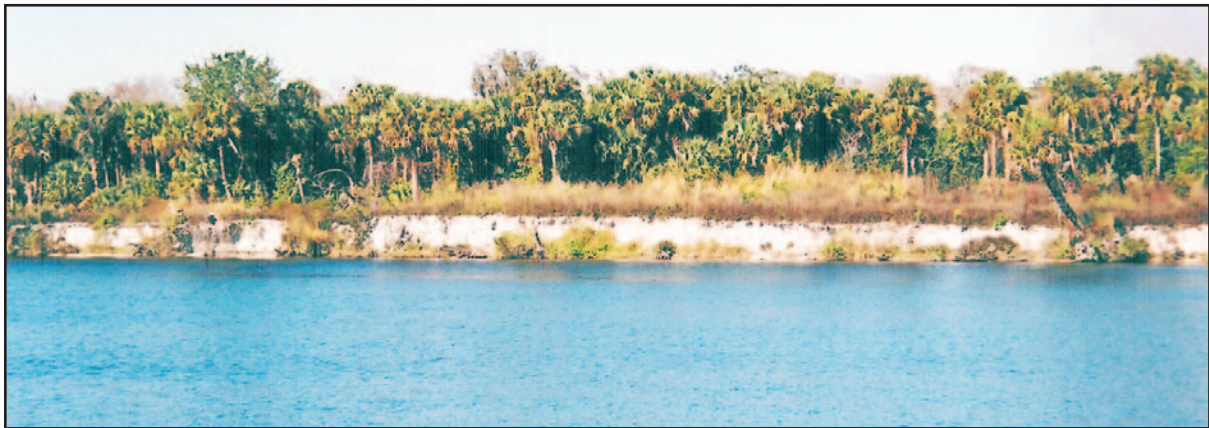
Figure 16. Side cast spoil along waterway at Rialto.
