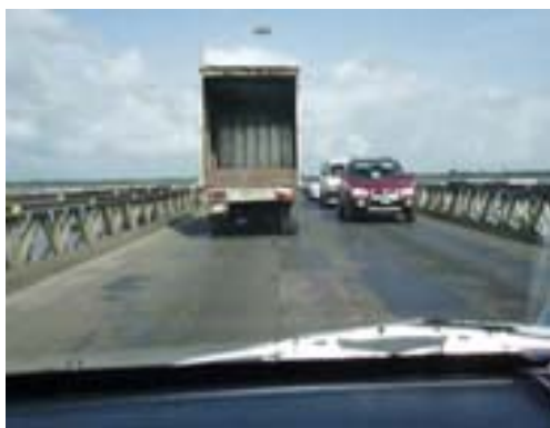
Photograph 1-2: Demerara Harbour Bridge aspects
