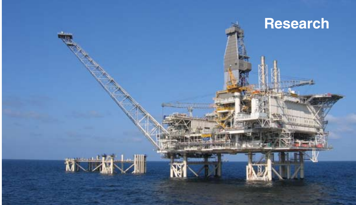
The newly constructed Central Azeri platform in the Caspian Sea will produce approximately 450,000 barrels of oil per day. The pillars to the left will support a platform for gas and water re-injection. Photograph courtesy of BP Azerbaijan.
