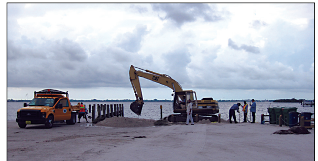
Sand shifting A work crew removes sand, part of a routine maintenance schedule, June 26 at the boat ramp on the Palma Sola Causeway, according to Seth Kohn of the city of Bradenton. The ramp and an adjacent parking lot at the southeast end of the causeway beach opened June 1. Islander Photo: Bonner Joy
