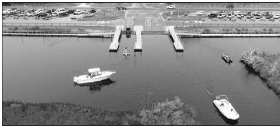
The project would include replacing the existing wooden docks with aluminum docks, along with six “finger” docks on each side.
