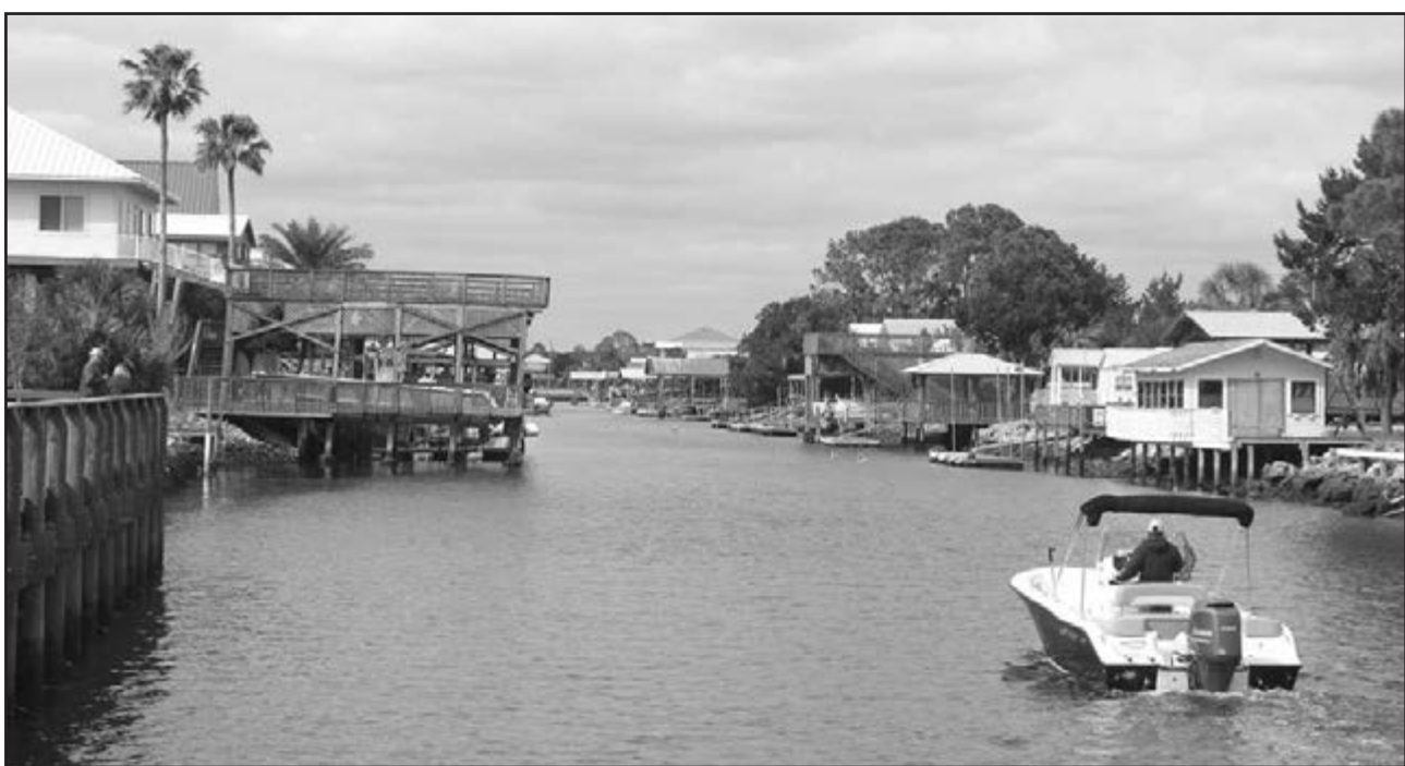
Canal dredging at Keaton Beach could begin this year, kicking off a string of dredging projects that could run through 2033, as the county moves next to Steinhatchee, Dark Island, Cedar Island and Dekle Beach.
