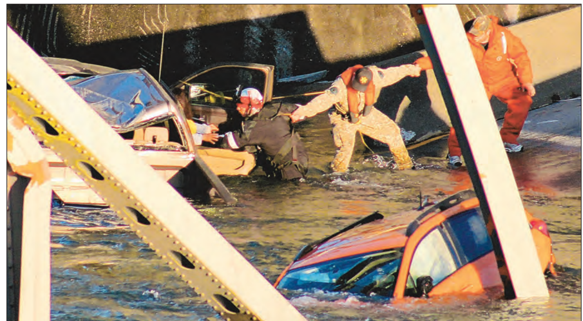
Associated Press Rescue workers form a human chain Thursday as they begin to remove a woman who reaches out from a smashed pickup truck that fell into the Skagit River after the collapse of the Interstate 5 bridge in Mount Vernon, Wash.
