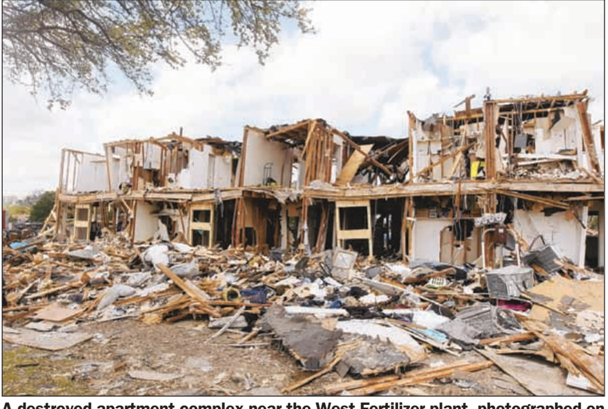
A destroyed apartment complex near the West Fertilizer plant, photographed on Sunday, four days after an explosion at the plant.
