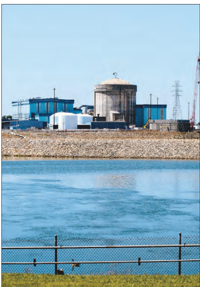
The working nuclear reactor is seen April 9, 2012, at V.C. Summer Nuclear Station in Jenkinsville, S.C.
