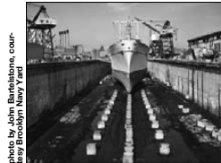
In Dry Dock 6 at the Brooklyn Navy Yard, tugs, barges, tankers and Coast Guard ships are still serviced and repaired.
