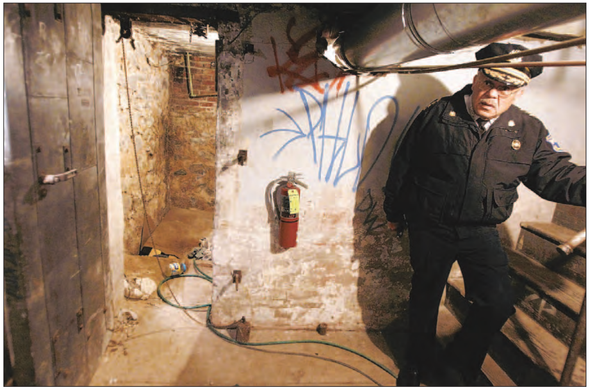
Associated Press Police Commissioner Charles Ramsey stands by the entrance Monday to the dank basement room in Philadelphia where four weak and malnourished mentally disabled adults, one chained to the boiler, were found locked inside over the weekend.
