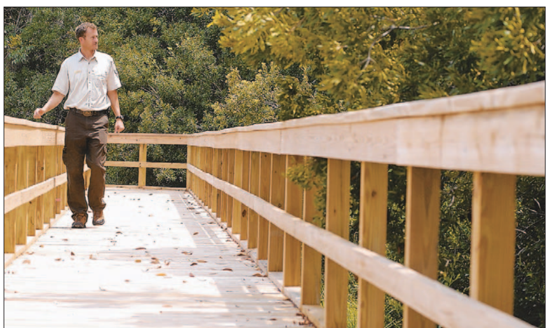
Boyd Blihovde walks along the new boardwalk. The structure is due to have finishing safety touches installed next week.
