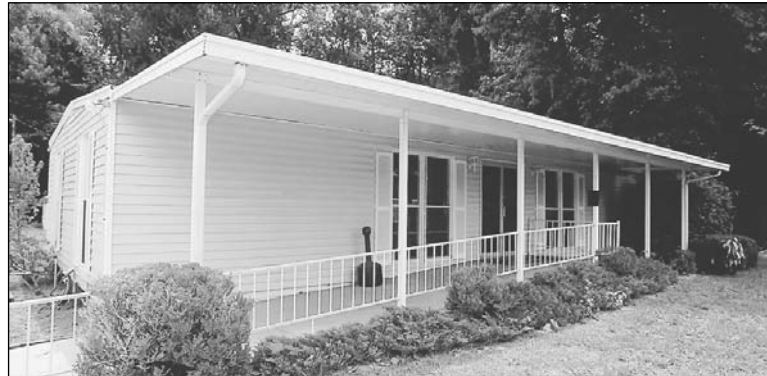
ABOVE: Suncoast Plumbing and Electric worker Frank Wells labors while renovating a bathroom in the new business incubator in Homosassa. BELOW: The former Homosassa Chamber of Commerce office is the new location for the business incubator.
