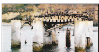
Abandoned wells Environmentalists: Tapped wells escape oversight./Page A10
