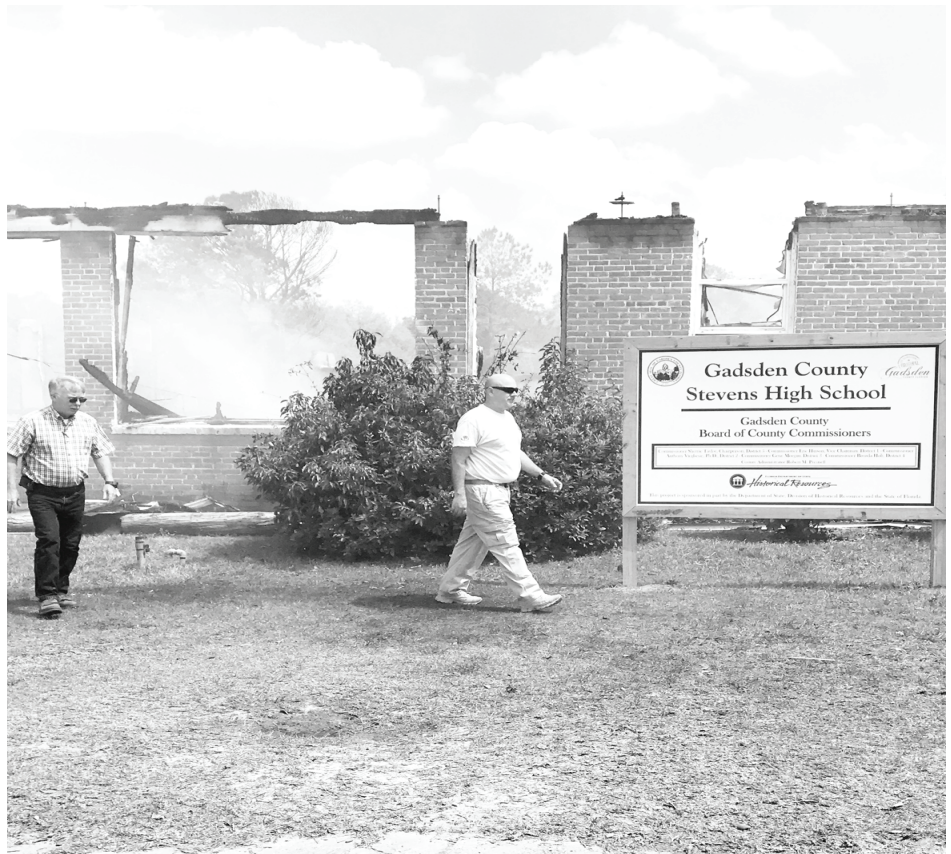
Also in March, the Old Stevens School was destroyed in a fire.
