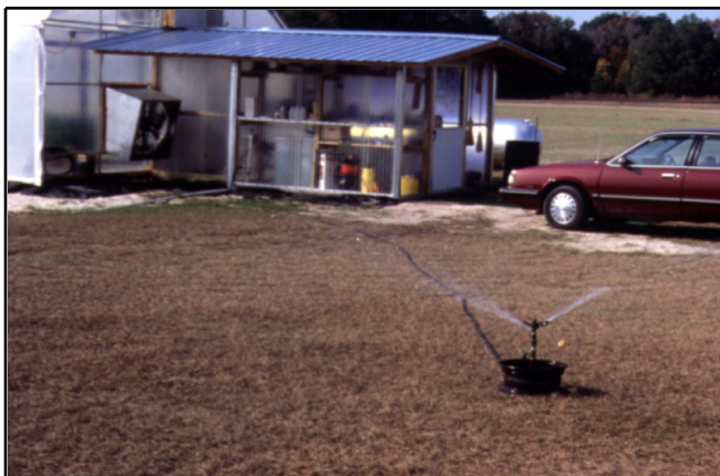
Figure 1. Airlock entrance room for sanitation control and work room.
