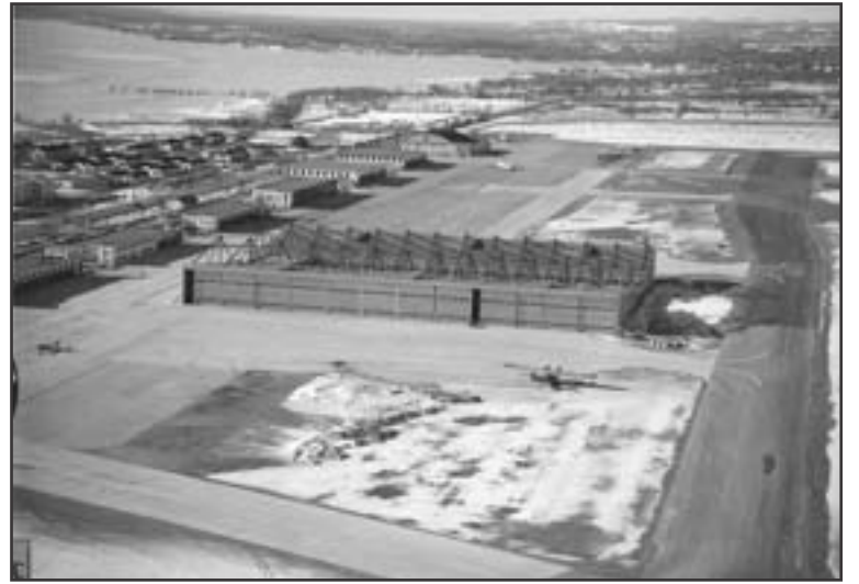
The new hangar at RCAF Station Trenton.
