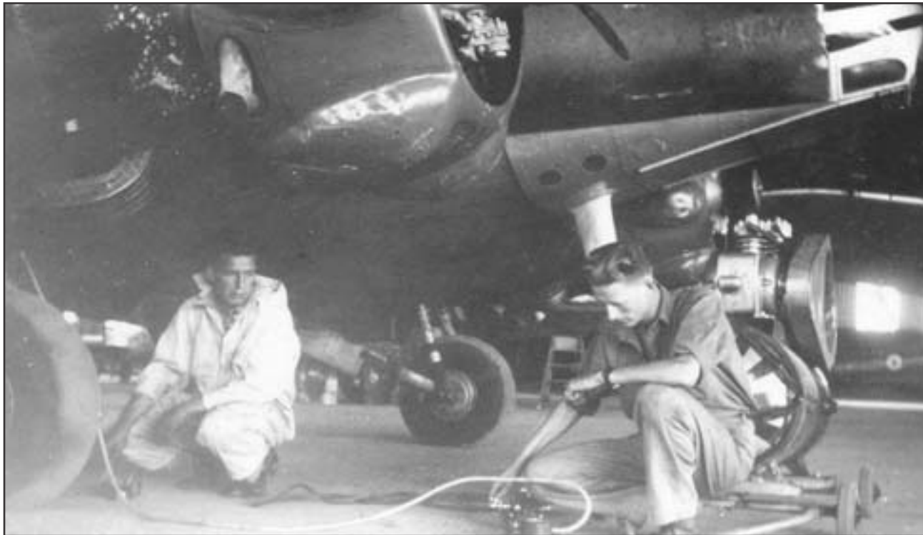
Maintainers inflate and check tire pressures on an unidentified BCATP aircraft, RCAF Station Trenton, Ontario. Circa 1944. Photo courtesy of the BCATP Museum, Brandon, Manitoba.
