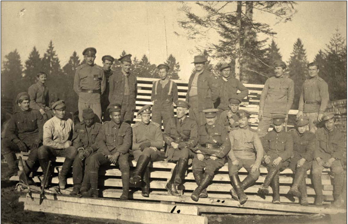
La Joux had men of various nationalities working there. Here, Russian soldiers are mingling with the men of No. 2 Construction Company and other military services.
