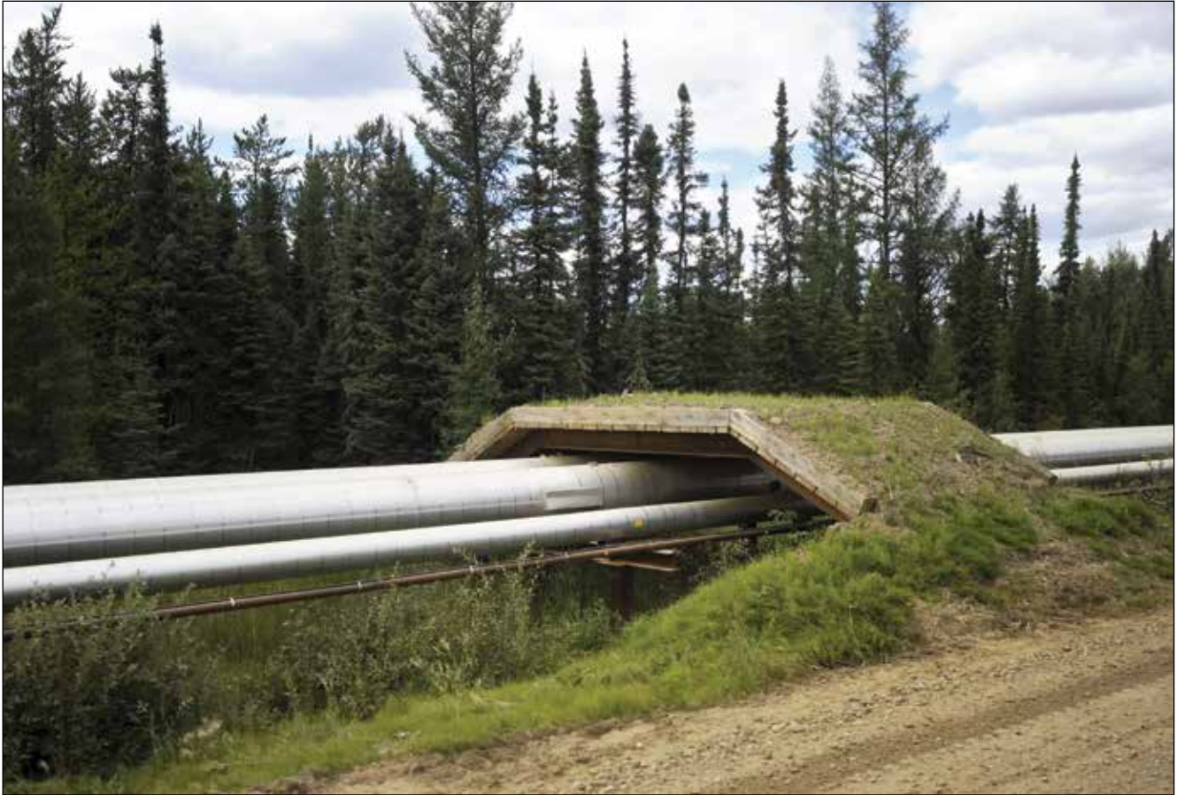
Wildlife crossing at Canadian Natural Resources Limited's (CNRL) Primrose Lake oil sands project is seen near Cold Lake, Alberta.
