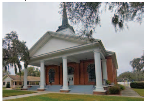
Photo by Steven Ryzewski The building for the First United Methodist Church of Fort Meade was built in 1911. The church community is celebrating its 150th anniversary.
