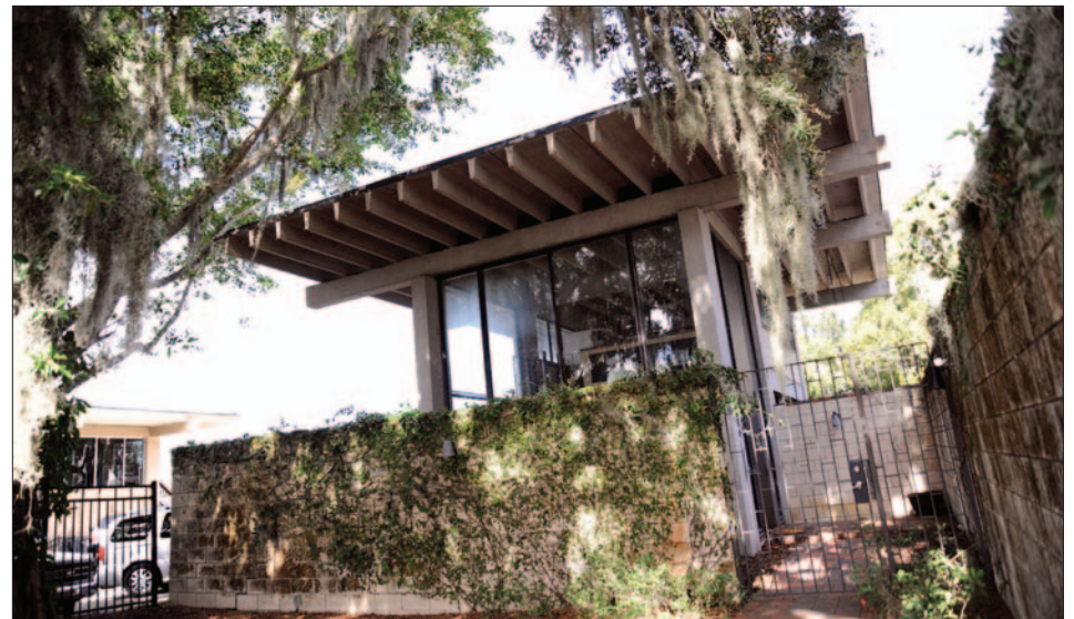
Gene Leedy built an office for himself in the style he is likely most famous for, concrete "double Ts" support structures, 8-inch overhangs, glass walls and black iron gates.
