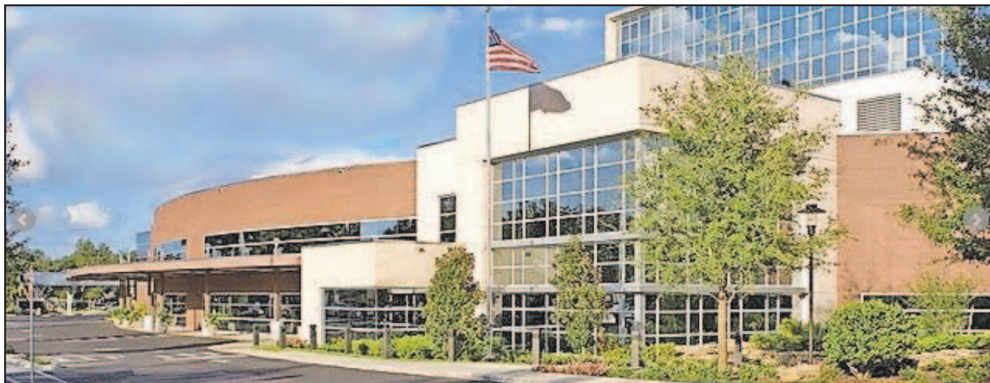
PHOTO PROVIDED Winter Haven Hospital today.
