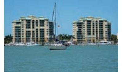
Pier 81 Condominium PH 2 Michelle Thomas 239.860.7176 Web ID 215018026 $1,595,000
