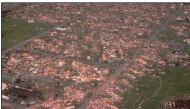
BOB EPSTEIN, FEMA NEWS PHOTO An aerial view of Miami-Dade County showing damage from one of the most destructive hurricanes in the history of the United States. Hurricane Andrew did extensive damage to homes in Miami, leaving little behind in its wake. One million people were evacuated and 54 died in this hurricane.
