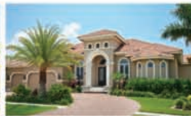
ROOKERY COURT ▲ Bay views from every room. Custom built in 2008. Pool/ spa, summer kitchen, 2 docks, 147' of waterfront. Furnished. $2,250,000 Brock/Julie Wilson | 595-5983
