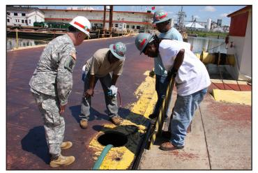
CH Wright, left, watches while Mat Sinking Unit (MSU) team members, left to right, Jimmy Grigsby, Austin Mayfield, and Walter McClure, pump water out to adjust the level of the barge to match the adjacent barge.
