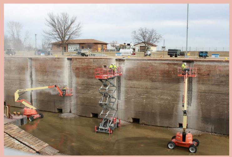
During the dewatering at Lock 17, crews accessed areas of the lock not normally exposed and repaired damaged portions of the concrete wall. *Photo by Samantha Heilig*
