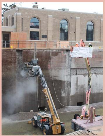
A hydro-demolition machine was used at Lock 17 to remove old concrete from the lock walls. *Photo by Samantha Heilig*
