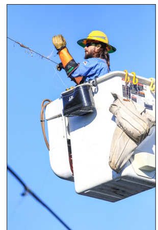
As a requested work order, Employees from the WREC removed fishing line that has been entangled on the powerline above the bridge where fishermen cast from on March 28, 2018
