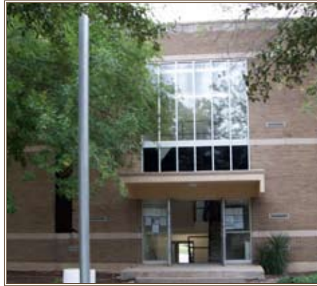
A brigade headquarters undergoes repairs thanks to the influx of ARRA funding Photos by William T. Harned, DPW, Fort Hood
