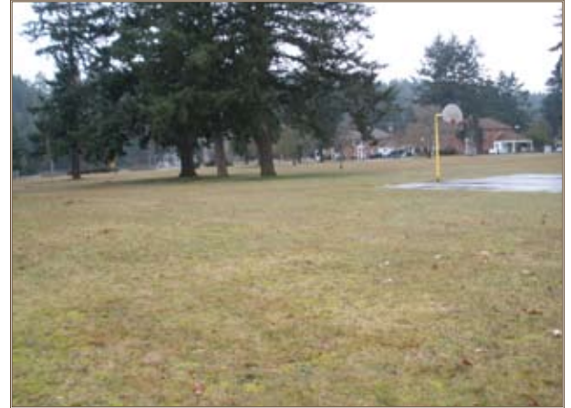
In just three months, Seattle District turned this four-acre bare property into a park that serves as a recreation site and memorial to Fort Lewis Soldiers killed in Overseas Contingency Operations. Photo courtesy of Fort Lewis
