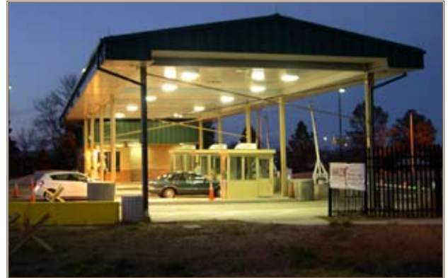
At Fort Carson, Colo., upgraded barriers and new guard booths are part of the ACP project. Photo by Gary Daniel
