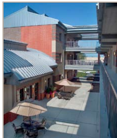
New dorms at Wright Patterson Air Force Base, Dayton, Ohio, Built by USACE, offer energy savings and elevated covered walkways help keep the elements away.
