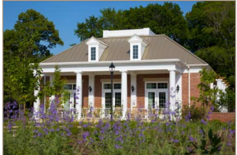
This Fort Belvoir neighborhood center earned LEED-NC Platinum certification. Photo courtesy of USGBC
