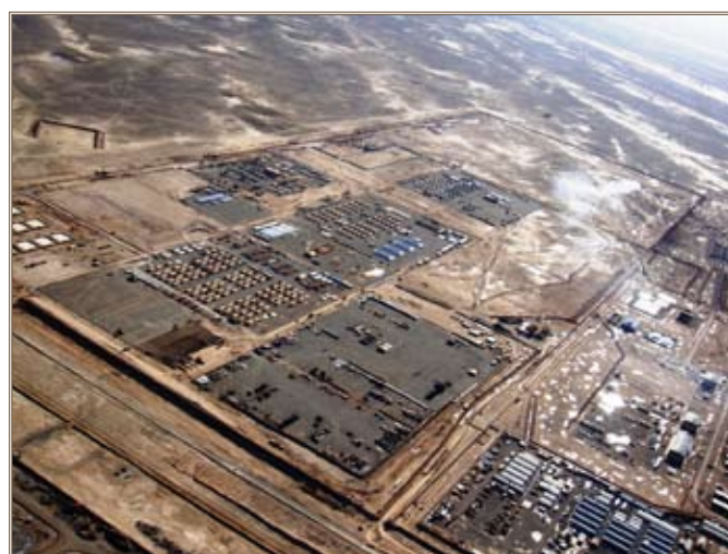
An aerial photo captures Forward Operating Base Leatherneck, Afghanistan, just after construction completion in April. The base, nestled on roughly 3,000 acres, was designed to support an initial population of 10,000 with a permanent population of 20,000 troops. U.S. Army photo
