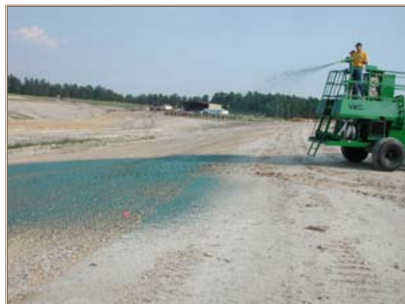
Land managers at Fort Bragg, N.C., apply a hydraulic erosion control product with a hydroseeder at the post's land-clearing and inert debris landfill. Engineer Research and Development Center photo
