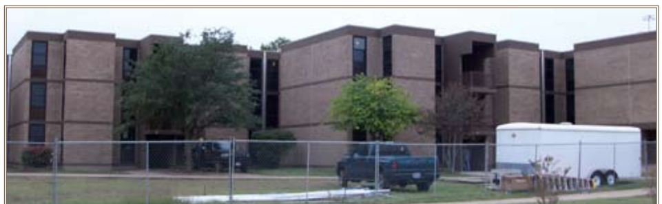
VOLAR barracks like this one will be renovated at Fort Hood as quality of life improvement for single Soldiers.
