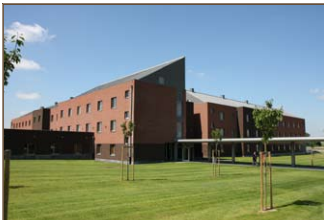
After 20 months of construction, the much-anticipated Army lodge opened on Chievres, Belgium, in June, replacing the leased Hotel Le Maisières and saving the Army close to $2 million a year. Photo by Justin Ward
