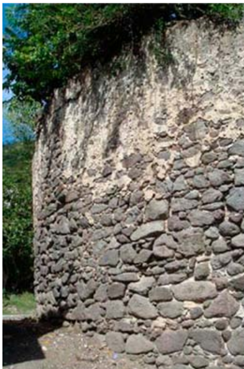
Figure 5. Exterior wall Airport Lime Kiln
