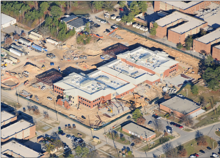
An aerial photo of the Quad DFAC while it's under construction.
