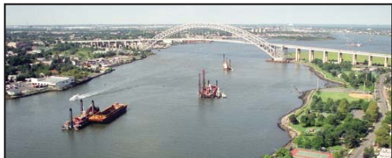
Three dredges work simultaneously in the Kill Van Kull near the Bayonne Bridge during deepening operations. (File Photo)
