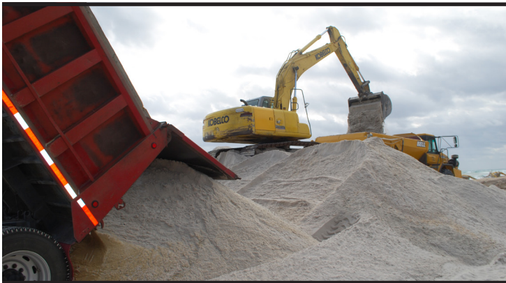
Contractors deliver sand to a beach access site where it's scooped onto off-road vehicles for distribution further down the beach. Like a well-oiled machine, contractors and Corps personnel oversaw the operations of more than 130 sand deliveries daily. (Photo by Susan Jackson)
