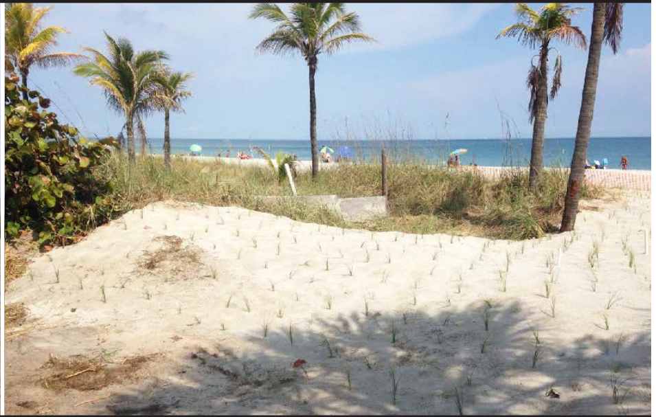
Before and after: Residents at the Starlight Towers complex temporarily relocated sea oats between the complex and the shoreline so the contractor could place sand in the low elevation area. Residents planted the vegetation to help protect the beach without realizing they cut off access for renourishment. (Photos courtesy of Eastman Aggregate Enterprises)
