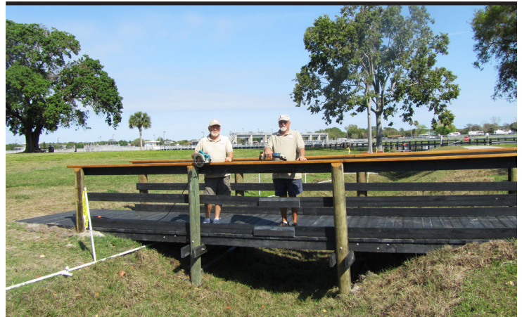
Volunteers George Schisler (left) and Donald Chapman (right) constructed this bridge using scrap composite material and lumber to provide safer, better access for the fishermen who use the recreation area.
