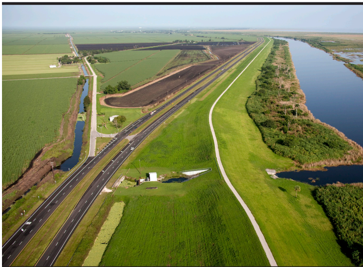
The Lake Okeechobee Scenic Trail (LOST) is on the crown of the Herbert Hoover Dike, which surrounds Lake Okeechobee. This section is near South Bay at the southernmost end of the lake. (Photo by Mark Bias)
