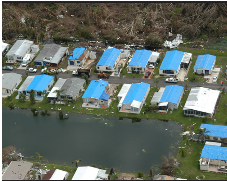
“Blue roofs” dot the landscape in this aerial photo taken near Port Charlotte following Hurricane Charley in 2004. Jacksonville District maintains Temporary Roofing and Temporary Housing Response Teams to assist local officials with unmet needs following a disaster. (USACE file photo)
